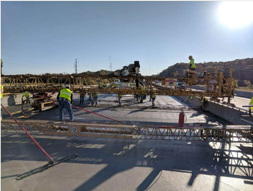
Phillips Hardy delivering innovation to bridge infrastructure with Helix Micro Rebar.
