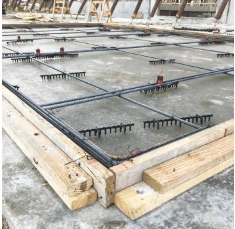
This thin panel has conventional reinforcing steel only at the perimeter and for the lifting inserts. TCA
