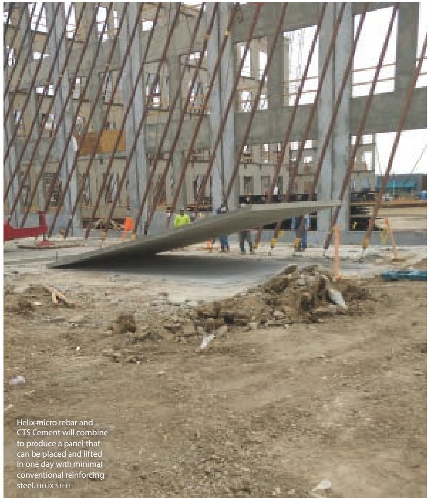
Helix micro rebar and CTS Cement will combine to produce a panel that can be placed and lifted in one day with minimal conventional reinforcing steel. HELIX STEEL
