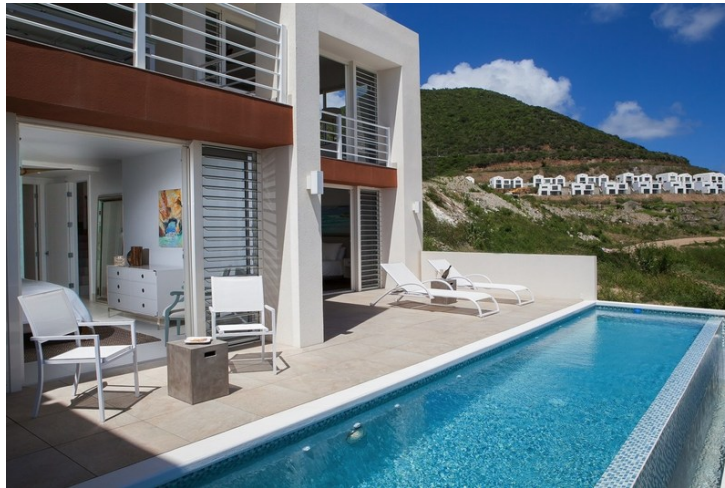
Helix Micro Rebar helps Indigo Green in Sint Maarten withstand a Category 5 Hurricane
